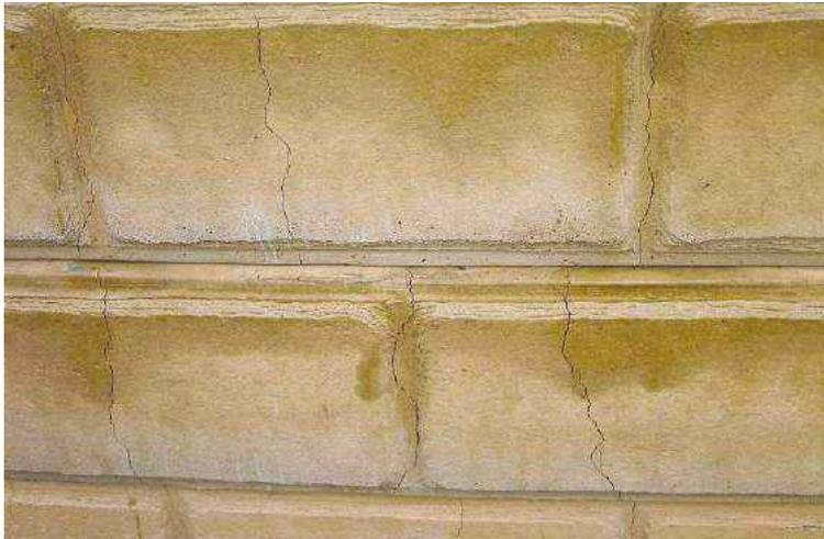
Stress fractures in concrete sleepers caused by heavy machinery drilling above the wall.
