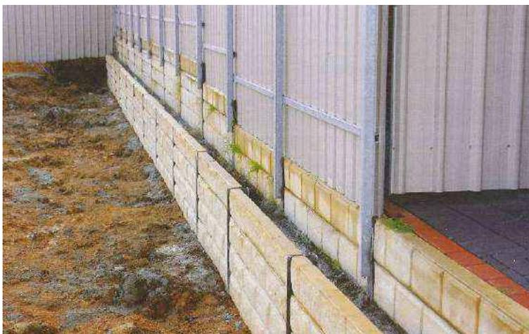
Completion of the undermined wall. Note concrete backfill used for increased stability.
