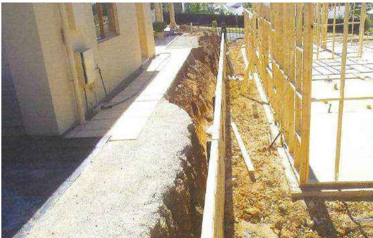
This wall was completed before studwork was erected. It would have been impossible to construct this wall after studwork due to restricted access.
