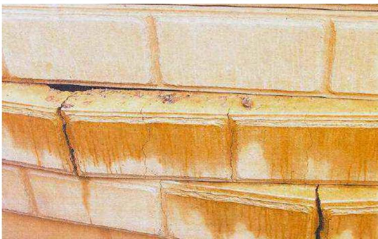
Backfill disaster due to material being pushed into the wall.
