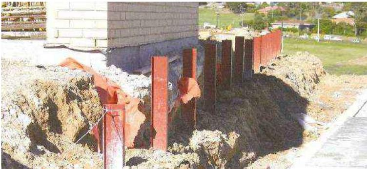
An example of a potential problem involving excavation and undermining. A joint wall would have been the better solution.
