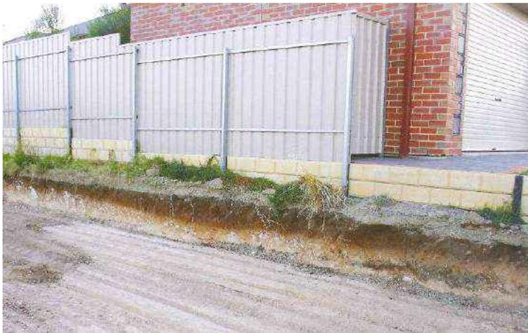
Note the excavation under the existing wall. Extra depth piers were allowed in the upper and as such there was no problem with undermining.
